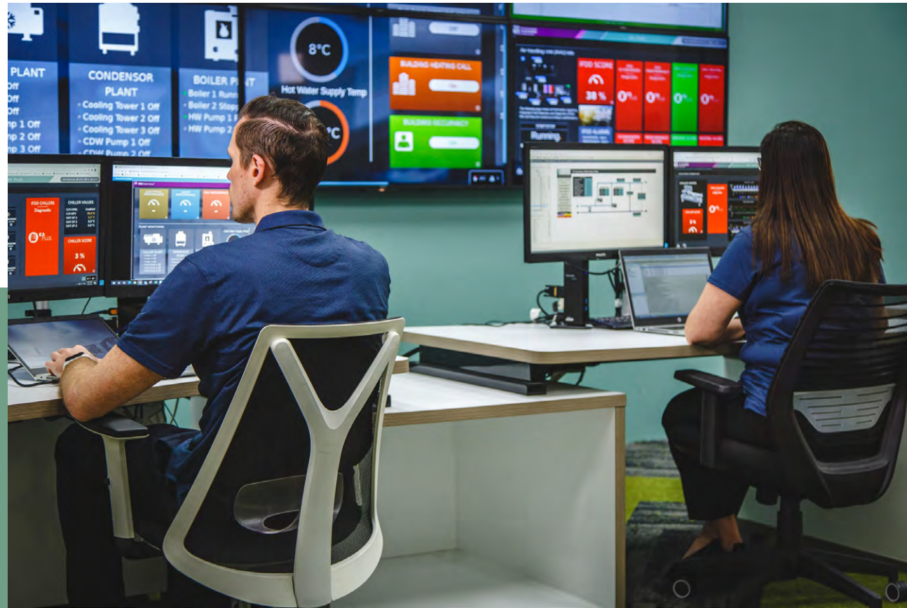
Environmental Automation's facility monitoring station equipped with RC-Reporter.
